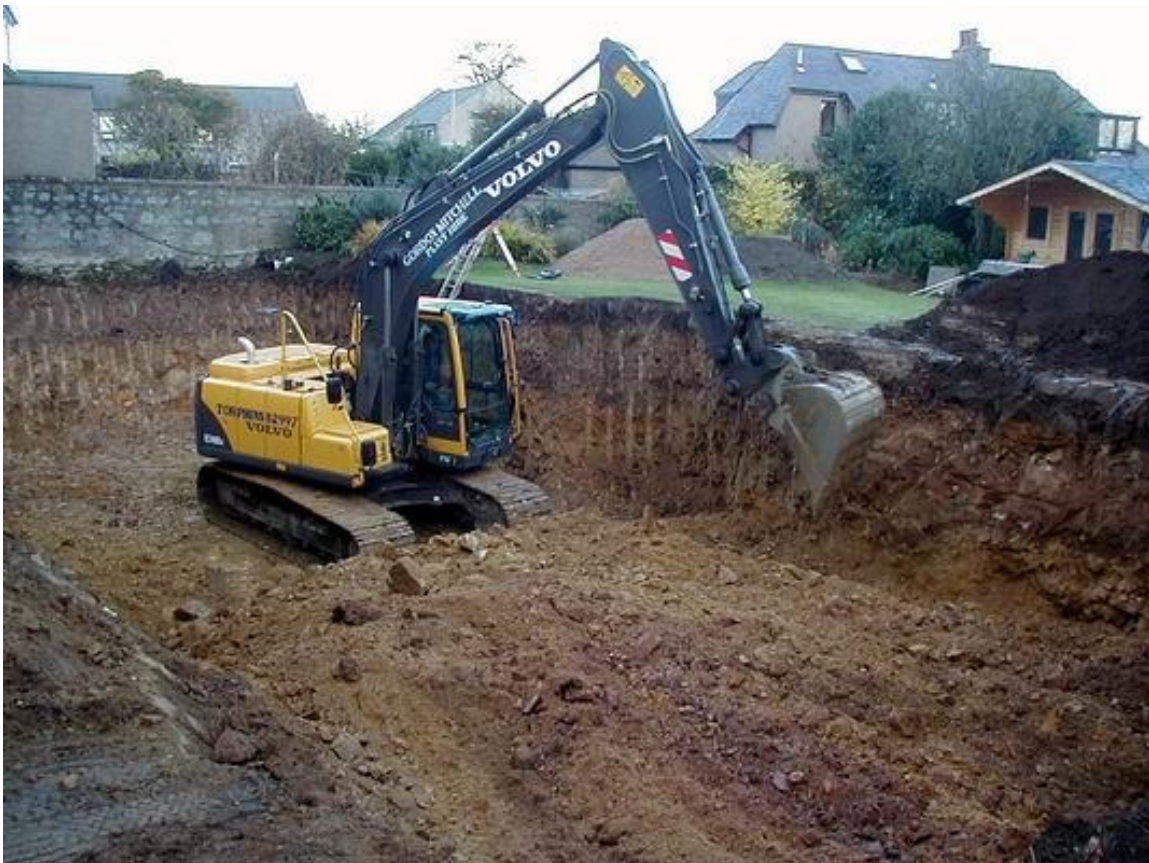
Digger in pit
